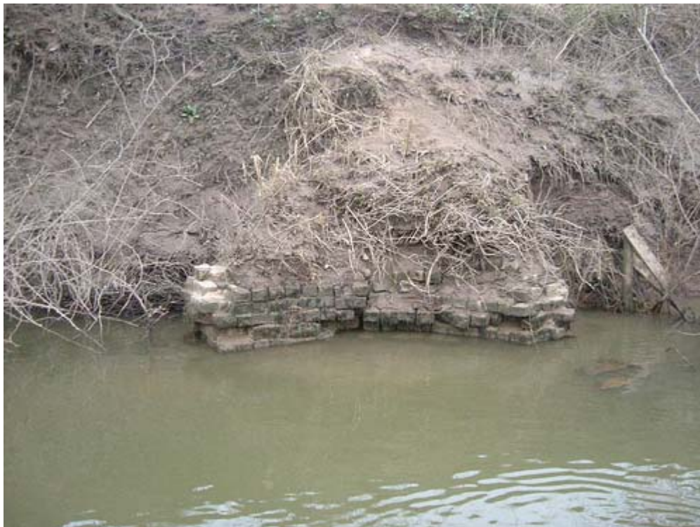
Brickwork visible under the river bank at Mythe Hooke
