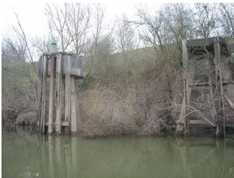
Timber towers below Upton-on-Severn for off-loading oil from river barges
